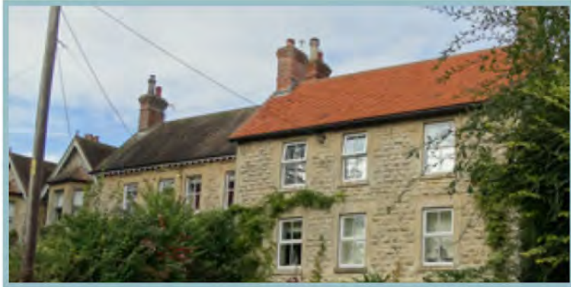
Gabled roofs with varying orientations. The left two has a street-facing double gable.
