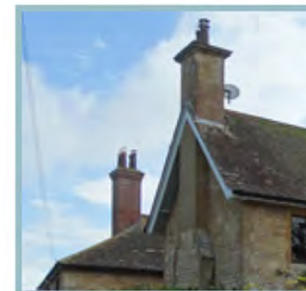
Stone chimney protruding from wall (front) and brick chimney stack (back).
