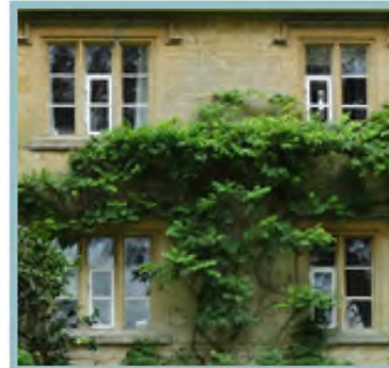
Casement window with chamfered stone mullions.
