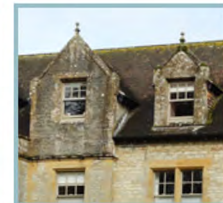
Gable wall dormer (left) and roof dormer (right) aligned with lower windows.
