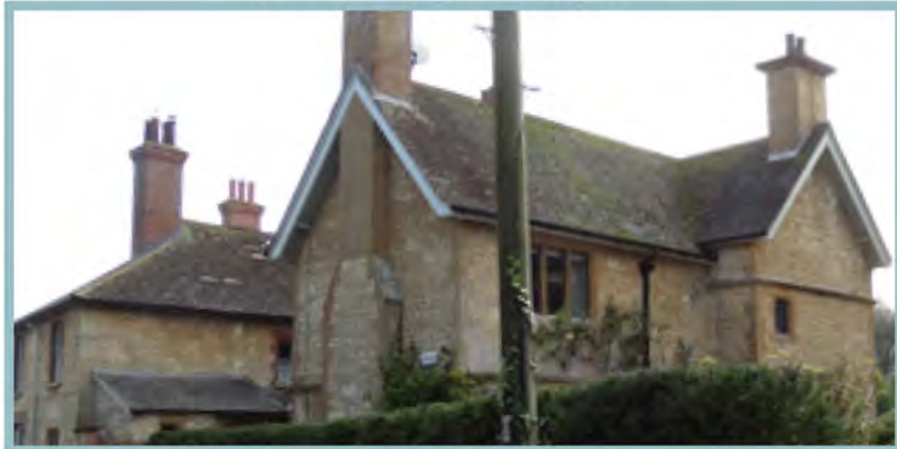
Crossed gable-roof (foreground) and hipped roof (background) with a lower projecting skillion roof.
