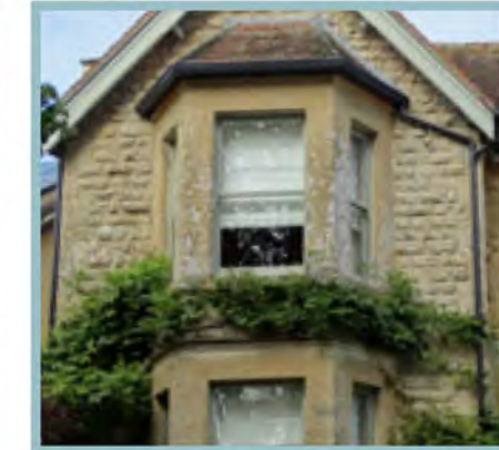
Double storey bay window with glazing set back into the walls to add relief.
