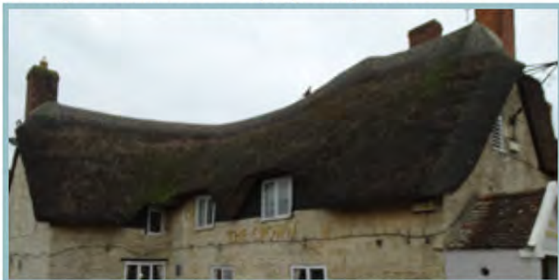
Crossed gable thatch roof with eyebrow dormers and a gable simple clay tile porch roof.
