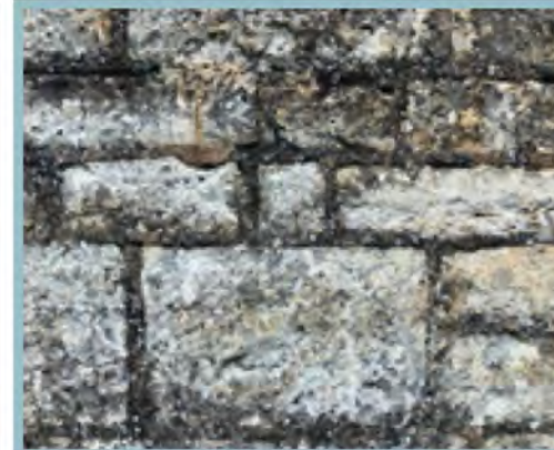
Rough course stone that has a darker hue than the Marnhull stone
