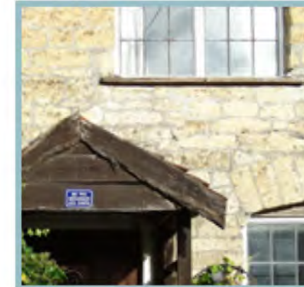
Natural wooden porch and fenestration with painted glazing bars.
