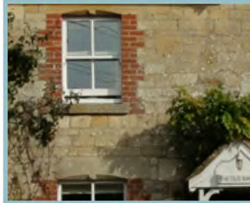
Semi-course Marnhull stone with limestone cill and brick dressing.
